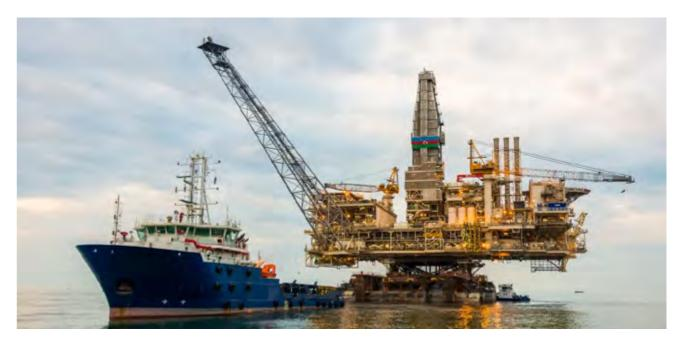
The \$6b project was announced following an agreement with the Government of Azerbaijan for extending the operational life of the ACG field until 2049. The project is designed to process 100,000 barrels each day of oil and 350 million standard cubic feet per day (Mscfd) of gas.
